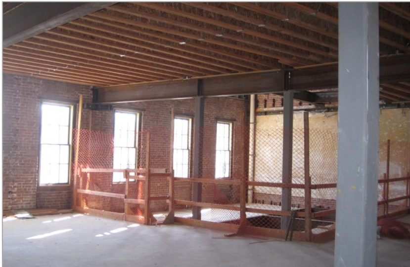
Existing Opening (Elevator Shaft)
